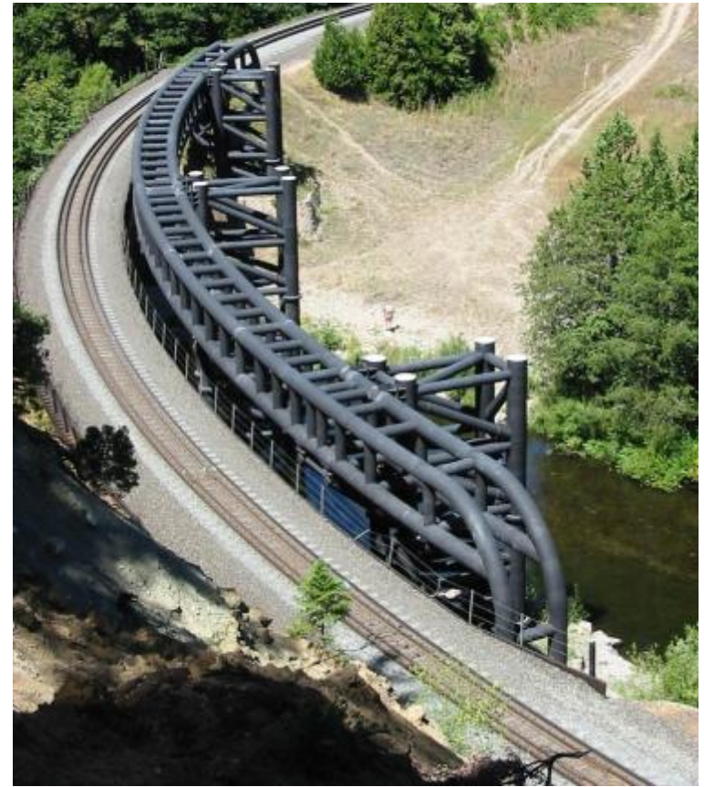
Bridge gaurd rail structure added to prevent rail cars from falling into the river.
